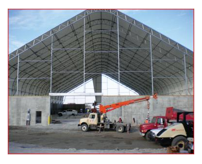
The salt dome repair scope of work for this project at M-4, M-5 & M-8 consisted of the removal and replacement of the existing asphalt shingle roofs, metal flashings & gutters, and the structural carpentry that was deteriorating. The existing interior and exterior light fixtures were removed and replaced with motion sensor LED light fixtures. The repair of these existing domes took place without shutting down ISTHA salt operations at any point.
