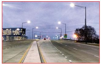
JBCC installed over 400 light poles with LED fixtures on Interstate 90 this past summer between Hoffman Estates to Rosemont, which totaled over 20 miles! In addition to the lights on I-90, JBCC installed new LED lights on the Meacham Road Bridge over I-90. This included new decorative light poles to improve bridge aesthetics and pedestrian friendly walkways over the Interstate.
